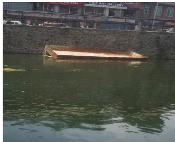
Fig. 2 Iron metal plate present at the Dal Lock Gate
